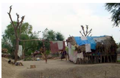
A house with poor roof construction Photo: CIET
