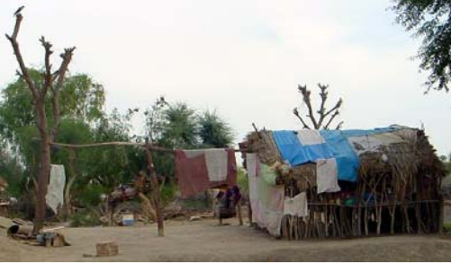
A house with poor roof construction Photo: CIET
